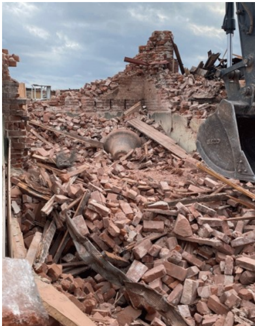
The bell of First Presbyterian Church in Mayfield was found in the rubble of the church building after it was destroyed by a Dec. 10 tornado. (Photo courtesy of First Presbyterian Church)
